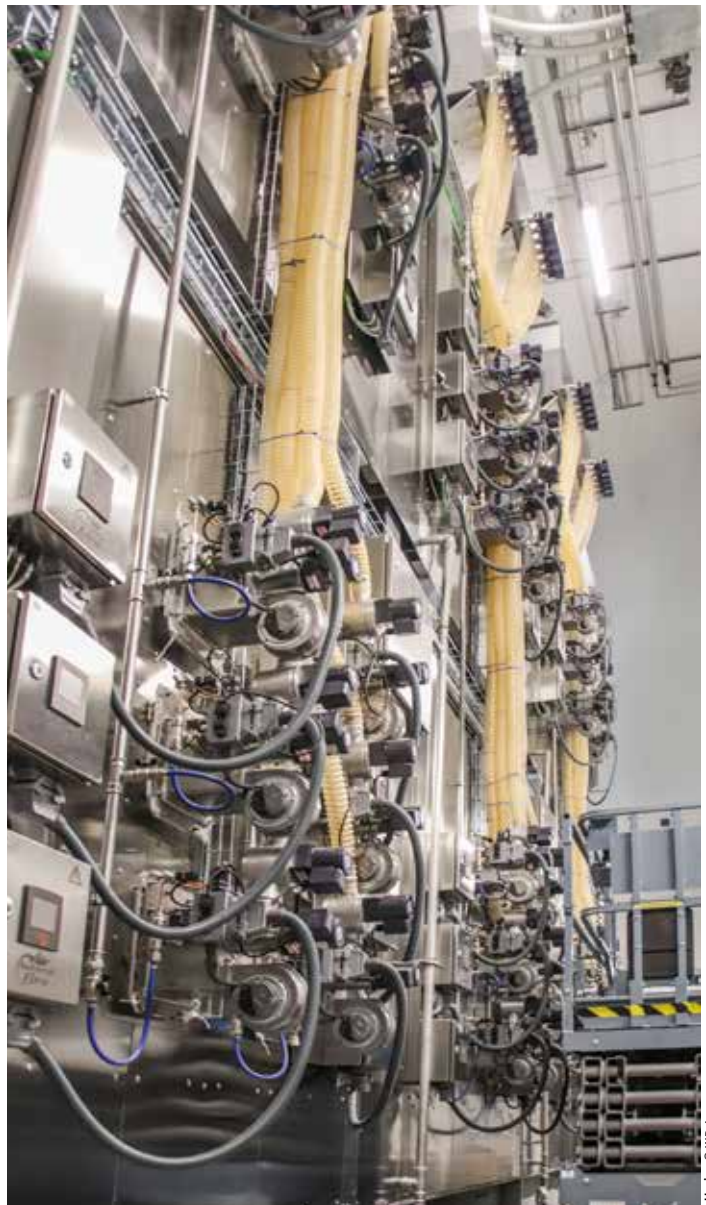
++ Rear view of the plant with pellet burners, control and automatic pellet feeding system
